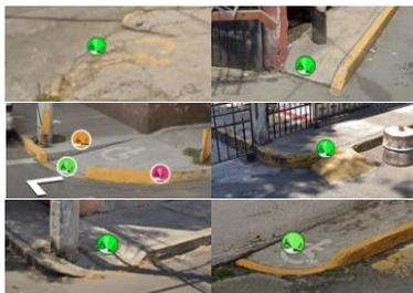
**Fig. 5:** Example curb ramps in Mexico rated as poor quality.
